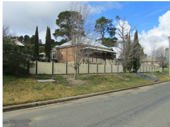
THE FORMER POLICE STATION
