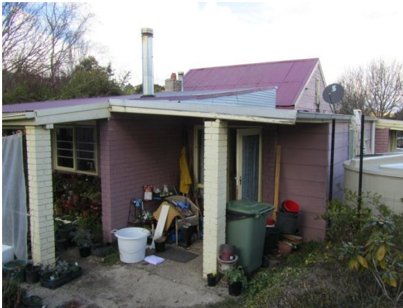
THE REAR/ NORTHERN ELEVATION
