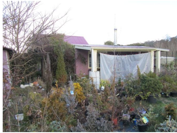
THE REAR/ NORTHERN ELEVATION
