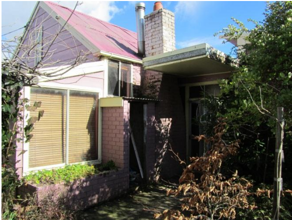
EASTERN ELEVATION VIEW, SHOWING THE GABLED ROOF OF THE ORIGINAL COTTAGE, INFILLED VERANDAH AND REAR WING
